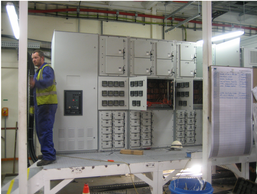
Figure 43: This photograph of part of the substation in the MICE hall clearly shows that a significant amount of electronics has been mounted in the front panels.
