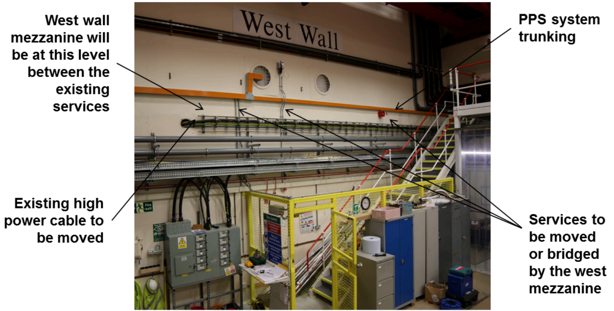
Figure 4: Current West Wall configuration.
